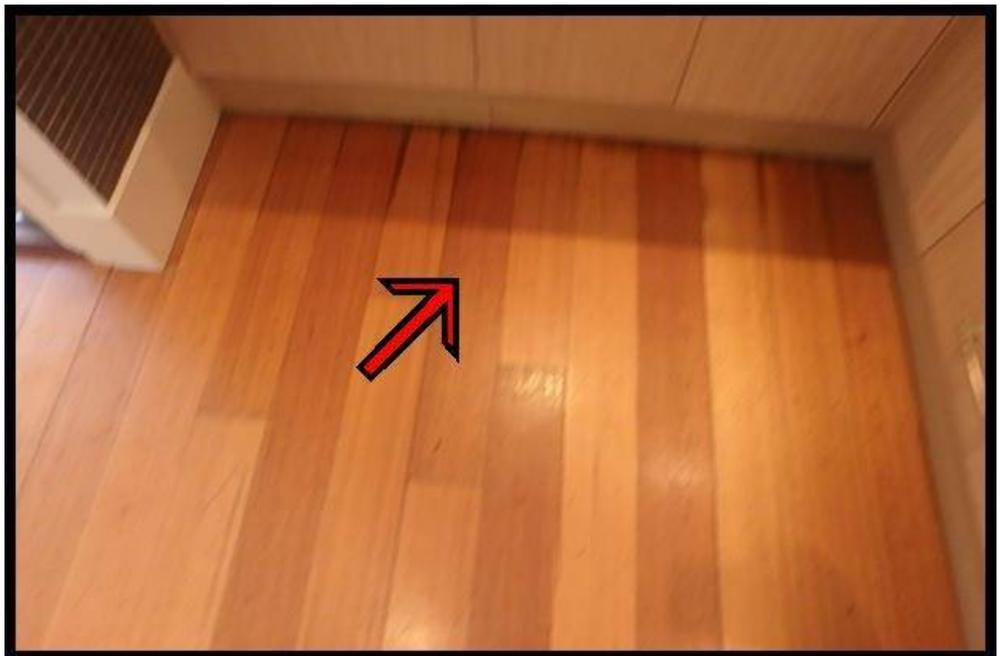
Tiles are not present to wet areas. Recommend tiles be installed to prevent water penetration.
